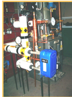
Customer heat exchanger (blue box)
